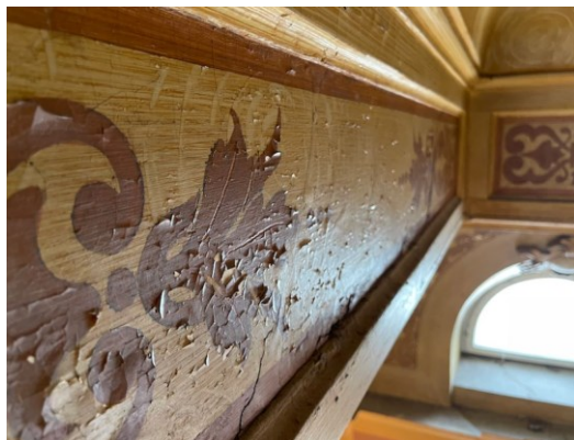
Fig. 4. The damaged wood texture imitation by means of painting. Photo by M. Paździora Sattler.
