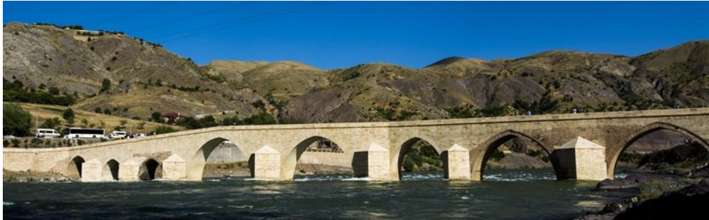
Fig. 6. Historical Palu Bridge
