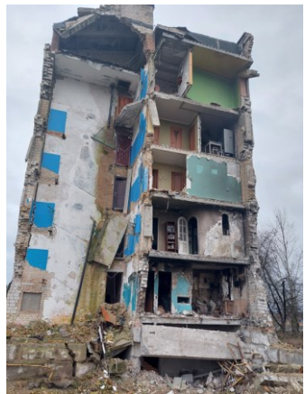
Fig. 7. A brick residential building with a floor made of precast hollow-core slabs at 429A Tsentralna Street after an air bomb hit. Photo by Y. Ivashko, 2023.
