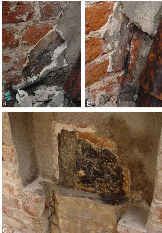
Fig. 8. Wrocław, Town Hall, southern façade: a. and b. remnants of plaster with traces of painted decoration above the roof of the eastern risalit (red, black and white); c. background of a niche in a buttress in the eastern part of the façade with traces of painted decoration (black)
