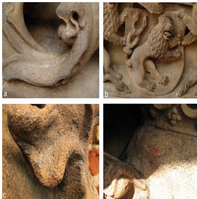
Fig. 7. Wrocław, Town Hall, southern façade, color remains: a. white and red paint layer on the tail of the griffin supporting the Silesian coat of arms; b. white monochrome on the lion in the coat of arms of the Kingdom of Bohemia and on the two lions supporting it; c. white monochrome on the surface of one of the griffin's labrums supporting the Jagiellonian coat of arms; d. red monochrome on the surface of the griffin's labrum supporting the Jagiellonian coat of arms
