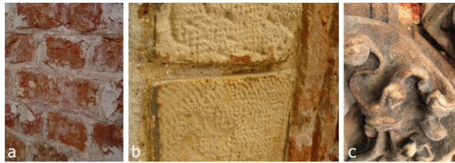
Fig. 6. Wrocław, Town Hall, southern façade, remains of colors: a. red monochrome on the joint and a brick surface; b. red monochrome on the stone block; c. red lead on the pinnacle
