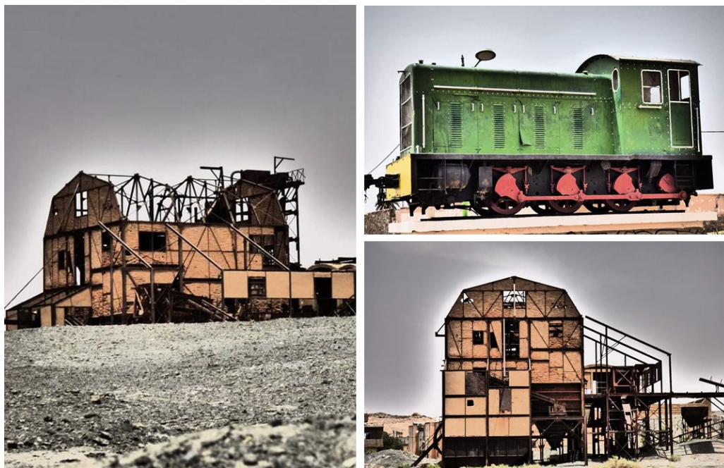
Fig. 4. Old industrial installations in Kenadsa
