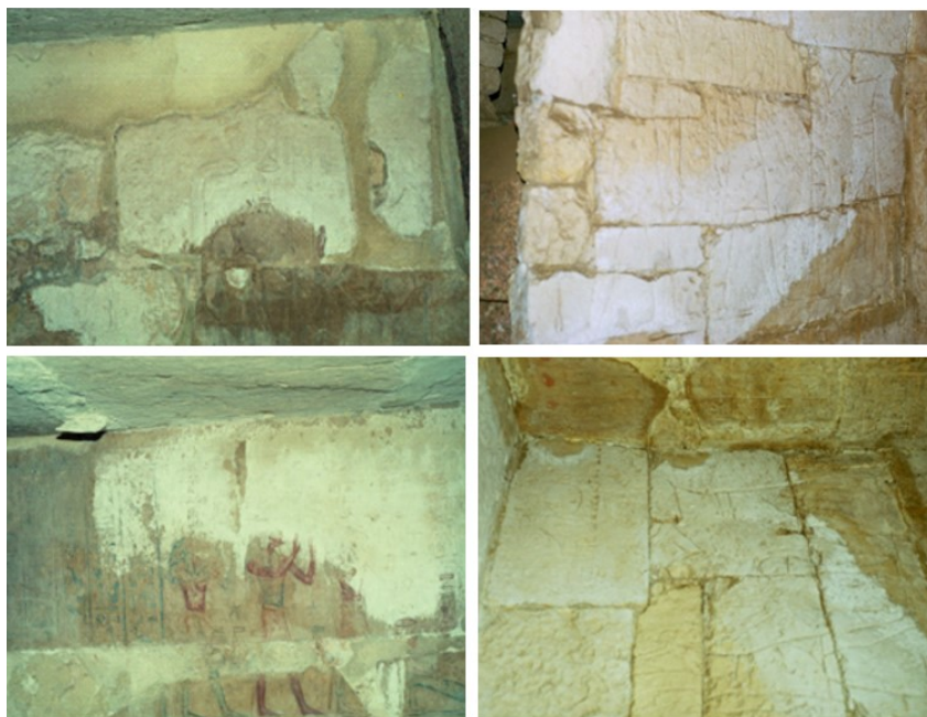
Fig. 4. The salt crystallizes thickly on the surfaces of the wall inscriptions in the royal tombs in San El-Hagar
