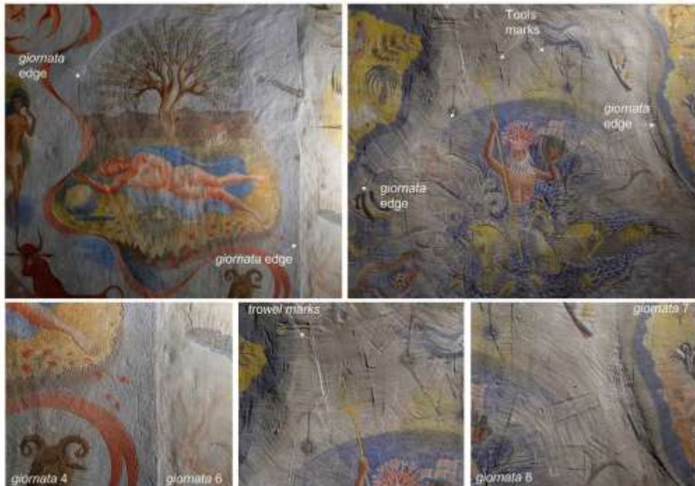
Fig. 3. On the top, Vis-Rak overview of plaster layout methods for giornate 1 to 6 (left) and giornate 6 to 8 (right). On the bottom, details where it can be seen the differences in the texture of the plaster between giornate , the different kind of joins and the marks of rectangle trowels used to lay and smooth the surface (photos by M. Ribeiro 2017. Project ALMADA).
