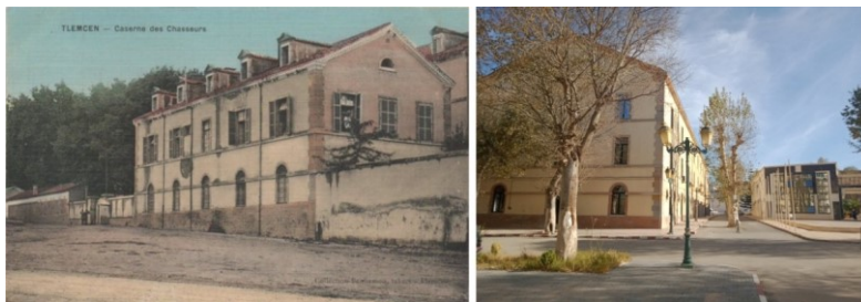
Fig. 5. The barracks of the African hunters during the French colonial period (left) [36]. The former barracks transformed into a medical faculty (right) 2022
