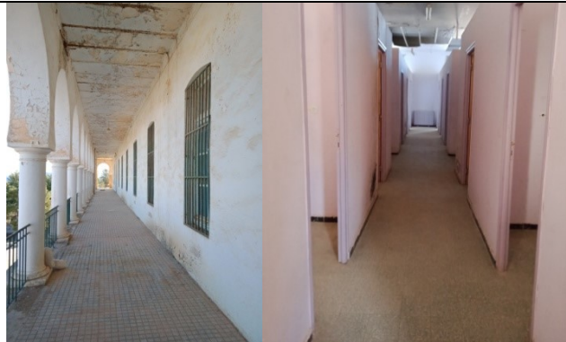
Views of the dormitory after the rehabilitation work
