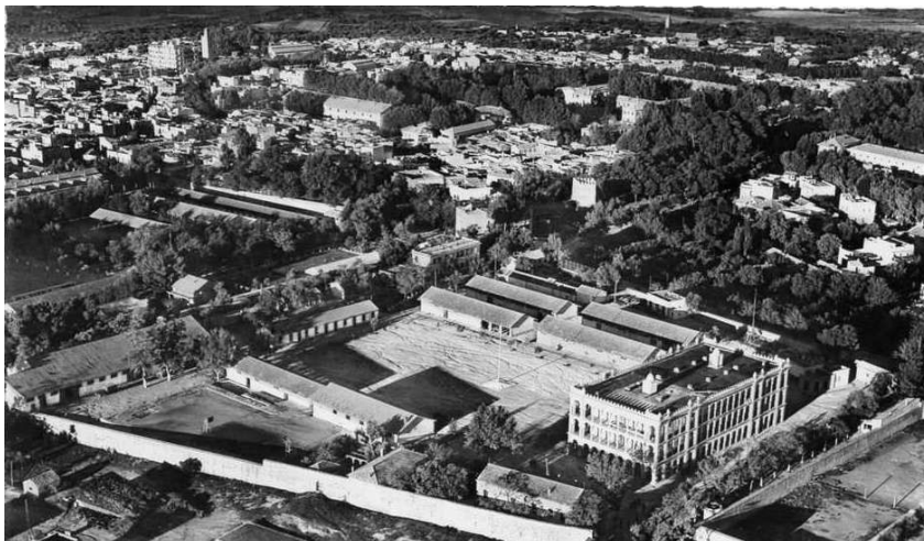
Fig. 8. General view of the Bedeau barracks after its construction [39]
