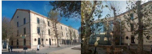
Views of the dormitory« block B» rehabilitated and converted into administration for the new faculty
