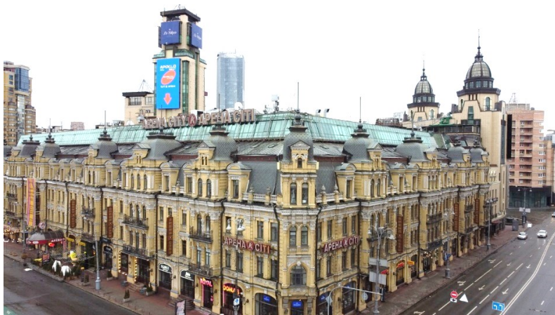
Fig. 1. The general appearance of the surveyed building. Photo by Oleksandr Molodid, 2021
