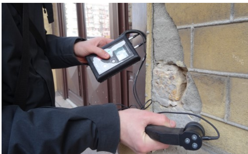
Fig. 4. The process of measuring the strength of stone facade structures. Photo by Oleksandr Molodid, 2021
