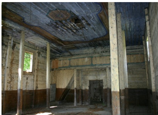
Fig. 5. Greek Catholic Church of the Dormition of the Mother of God in Babice; interior from the side of the choir, visible division into pseudo-aisles obtained with the help of the rows of pillars; photo T. Tomaszek
