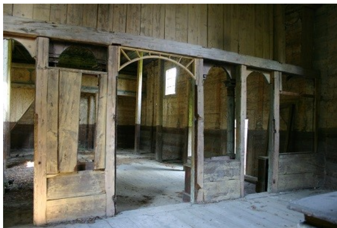
Fig. 21. Greek Catholic Church in Babice – the frame of the iconostasis with elements of woodcarving (view on the back, i.e., from the side of the sanctuary), photo T. Tomaszek
