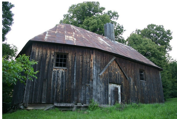
Fig. 3. Greek Catholic Church of the Dormition of the Mother of God in Babice; view from the north – traces of a lost sacristy on the wall; photo T. Tomaszek
