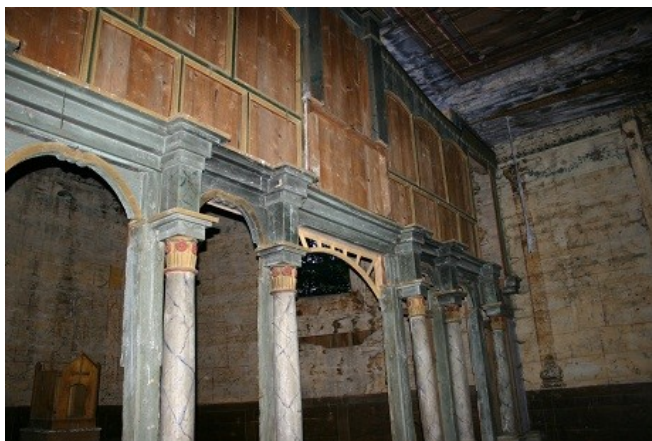
Fig. 20. The Greek Catholic in Babice - the frame of the iconostasis with elements of woodcarving (fragment) constituting the remains of the original equipment of the temple (and at the same time serving as a structural "curtain wall" separating the sanctuary from the nave), photo T. Tomaszek
