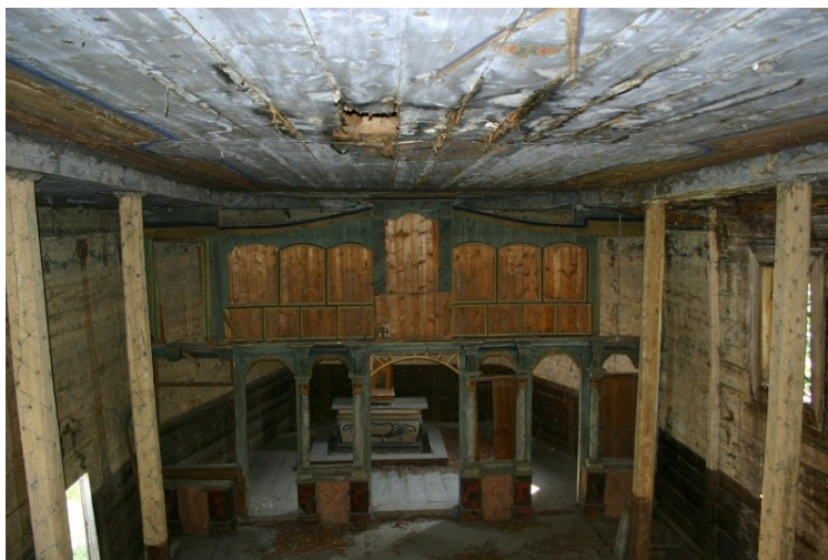
Fig. 17. The Greek Catholic Church in Babice – the iconostasis curtain wall without icons, which is separating the sanctuary from the nave, photo T. Tomaszek
