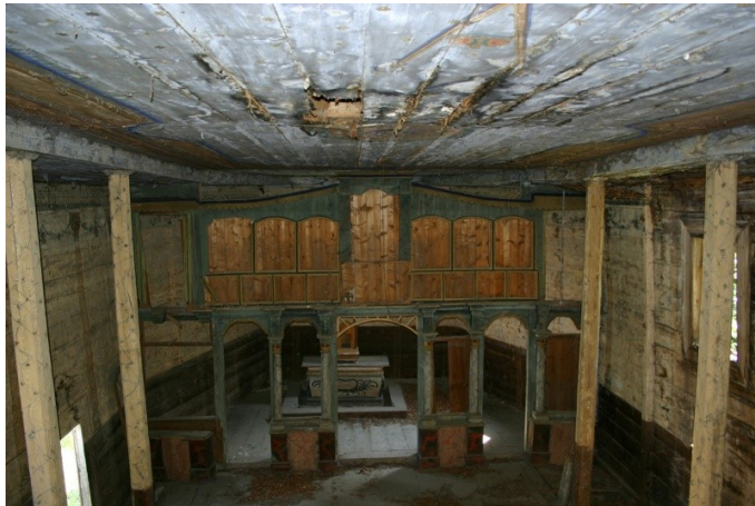
Fig. 6. Greek Catholic Church of the Dormition of the Mother of God in Babice - view of the sanctuary separated from the nave by a curtain wall of iconostasis (currently devoid of icons), photo T. Tomaszek.
