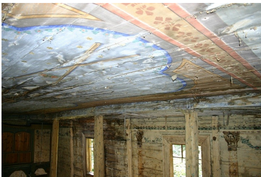
Fig. 13. Greek Catholic Church of the Dormition of the Mother of God in Babice - ornamental polychrome covering the walls and imitating architectural divisions, currently in very poor condition - view of the southern wall of the nave and the sanctuary (iconostasis wall), photo T. Tomaszek
