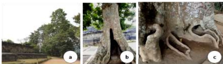
Fig. 8. a. An old Canarium vulgare tree grown very close to the Borobudur temple; b. Large cavity with decayed tissue in the stem base of Canarium vulgare ; c. The basal area of Canarium vulgare with tissue damaged symptoms.
