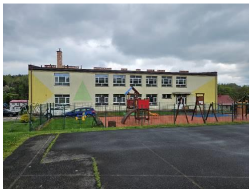
Fig. 2. Primary School in Bezmiechowa Dolna
