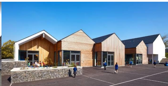
Fig. 5. Kirkmichael Primary School / Holmes Miller Author: Andrew Lee https://www.archdaily.com/570044/kirkmichael-primary-school-holmes-miller/546eb6f9e58ece1d3600012a-2706_kirkmichael_ps_8-jpg?next_project=no
