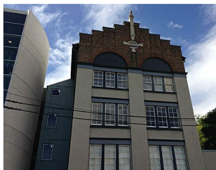
Fig. 9. International Grammar School - 2012 End of Year Works https://www.greenpointgroup.com.au/projects/education/item/64-international-grammar-school-2012-end-of-year-works Author: Greenpoint Construction Group Pty Ltd
