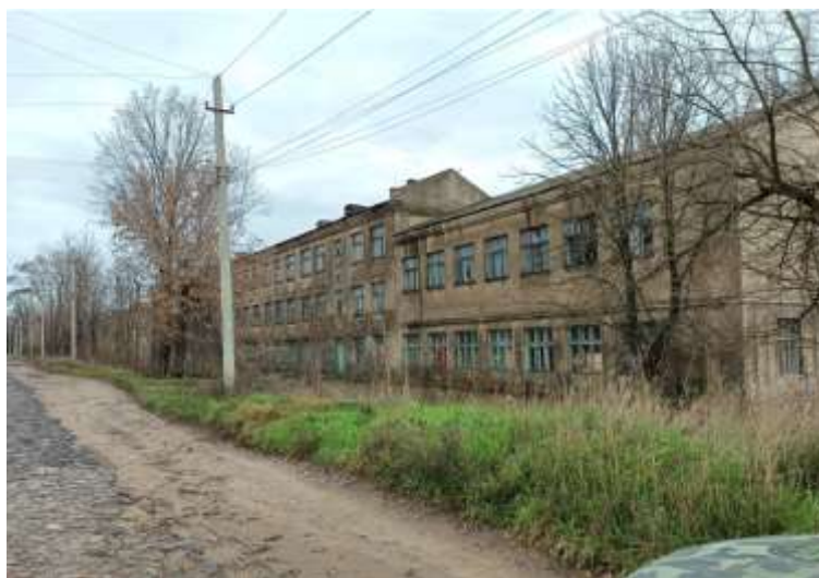
Fig. 1. Buildings of the industrial enterprise in Bakhmut (Donetsk region).
