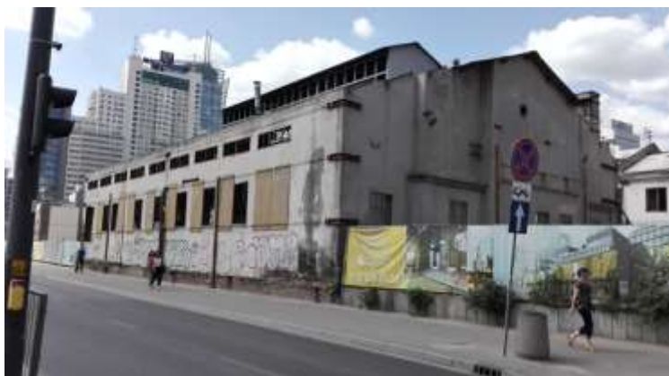
Fig. 4. One of the "Fabryka Norblina" buildings in the process of revitalization.
