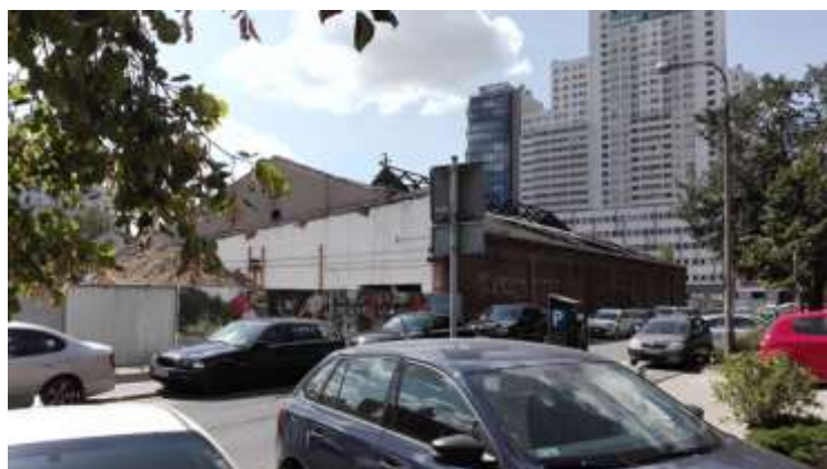
Fig. 5. The "Fabryka Norblina" plot is in the process of reconstruction.
