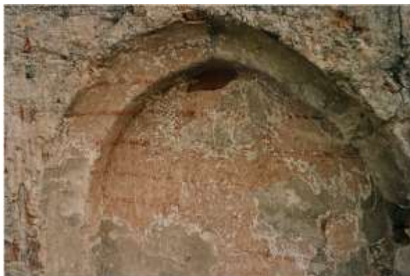
Fig. 11. Namysłów, south elevation of the town hall, fragment of an ogival recess with a painted imitation of bricks, photo by the authors
