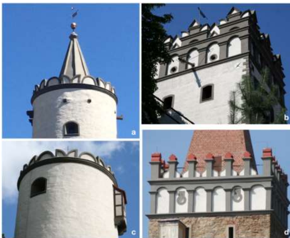
Fig. 7. Attics of the gate towers: (a) Paczków, the tower of Kłodzko Gate (mid-16th century), (b) Grodków, Lewińska Gate (around 1600), (c) Paczków, the tower of Ząbkowice Gate (mid-16th century), (d) Głuchołazy, the tower of Upper Gate (around 1601)
