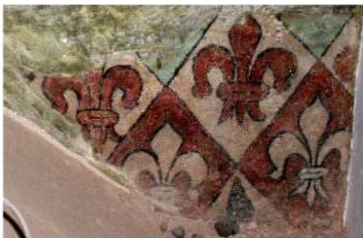
Fig. 15. Wrocław, the tenement house at Rynek 6. The remains of the polychrome with Boners' lilies that survived in the vaulted groins under the floor of the first storey; state during the renovation of the tenement house in 2008, photo by Agnieszka Gryglewska n) (used with permission)
