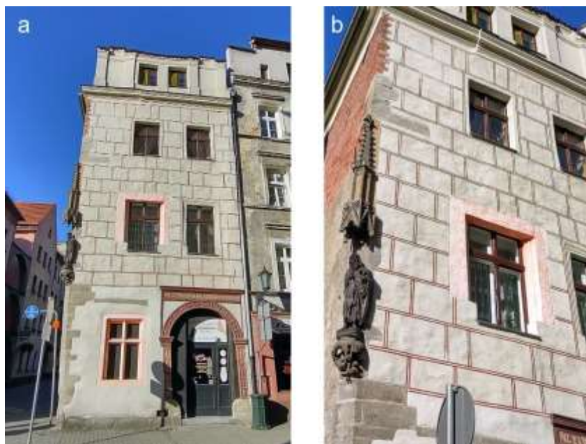
Fig. 10. Świdnica: (a) medieval tenement house in the corner of the market square and No.2 Łukowa Street, (b) view of the facade, which was covered with bright plaster in the 16th century, and on which the illusion of stone cladding was painted with red stripes, photo by the authors
