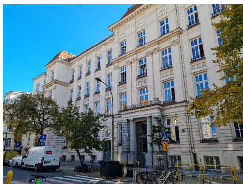
Fig. 10. View of the front façade of the building of the 20th Secondary School from the semi-western side, October 2022
