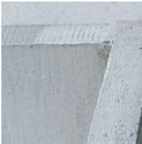
**Fig. 17.** Infill housing development - a residential building right corner, dating back to 1961 at 28 Czerwca 1956 nr 138. A study of stone damage due to the use of improper facade paint. No possibility of air reaching the structure of the material.
