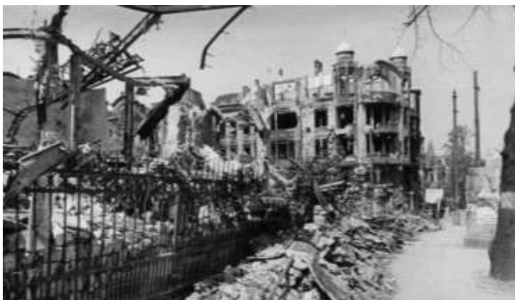
Fig. 7. Residential buildings destroyed as a result of the war, Roosevelt street in Jeżyce, the second half of the 1940s. Source: Sakson, Skarzyński 2008
