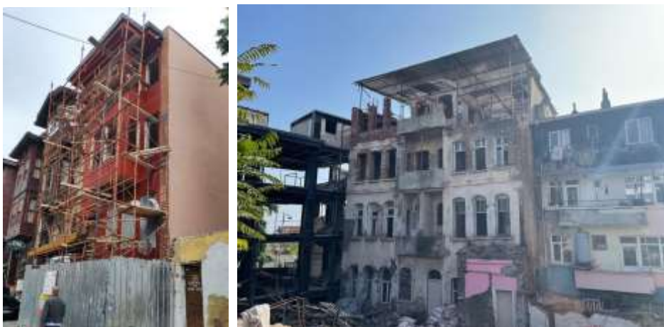
Fig. 2. The examples of masonry civil architectural structures in Fatih area: poor work cage (left) and people working without proper work precautions (right)
