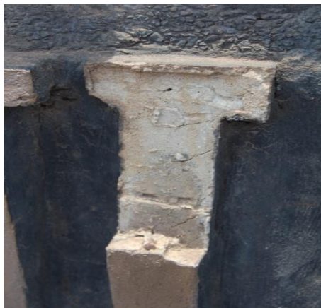
Fig. 4. Break offs on the pedestal of the sculpture
