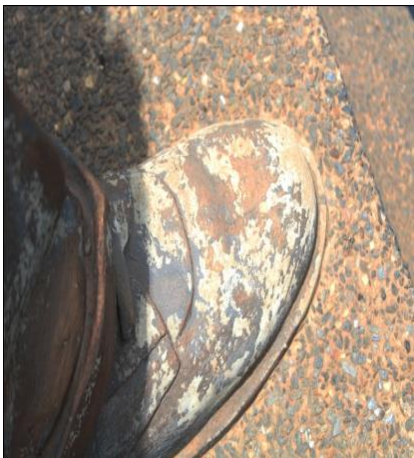
Fig. 1. Fading and peeling of paint on the sculpture
