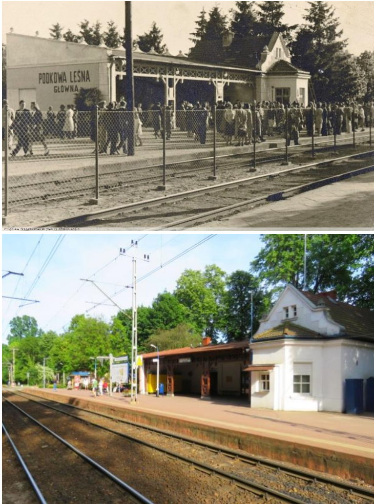
Fig. 9. Railway station in Podkowa Leśna from 1927 [26]
