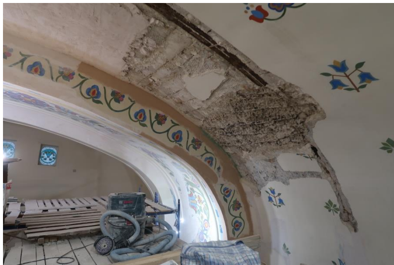
Fig. 6. Repair process of the vault surface. Photo by P. Baiandin, 2022.
