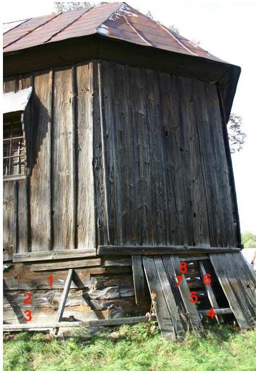
Fig. 4. The Orthodox Church in Miękiszy Stary. Sanctuary (south-east corner) – the spots were Resistance Drilling analysis were carried out shown by corresponding white arrows with numbers
