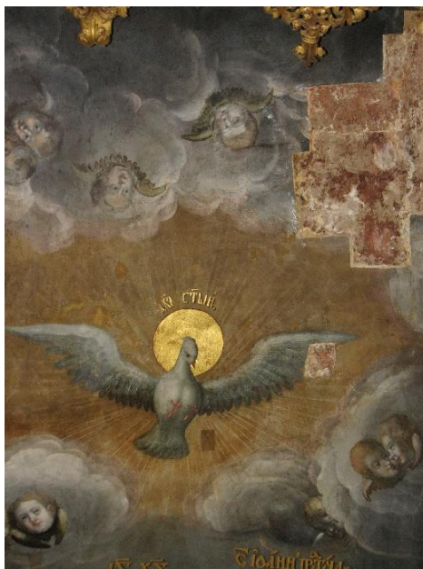
Fig. 3. Probe with the disclosure of the remnants of the adhesive painting on the composition of the southern vault of the transept
