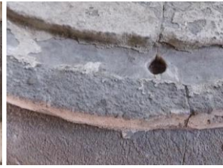
Fig. 20. Furrows in the direction of water flow, the result of crystalline mass dissolution
