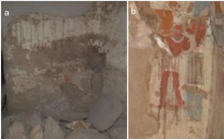
**Fig. 10** a - infiltration of rain and wastewater by ingress through cracks; b - discoloration in appearance due to the prolonged action of microorganisms
