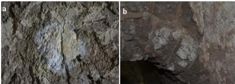
**Fig. 7** a, b - accumulation of soluble salts at the mudbrick
