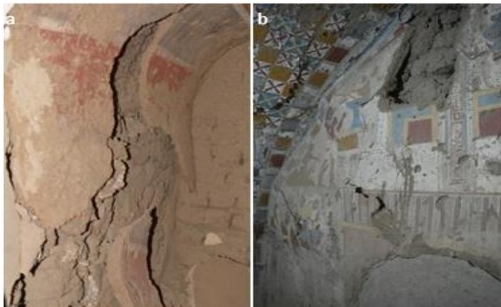
**Fig. 4.** a - Displacement, leaning of the wall:
