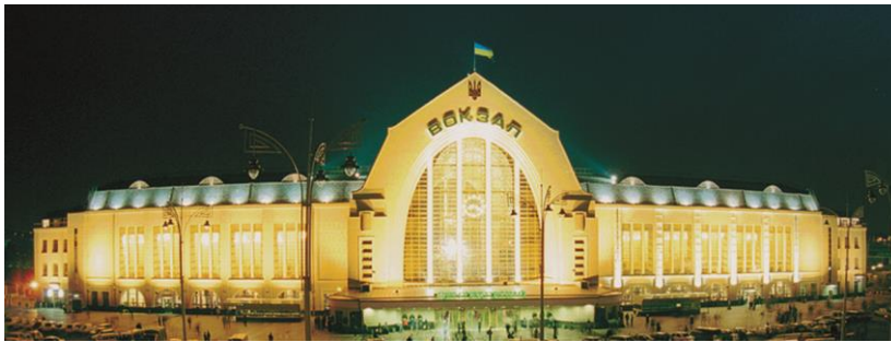
Fig. 3. Main facade of the station building after restoration. Photo from the funds of the Ukrrestavratsiia corporation, 2020
