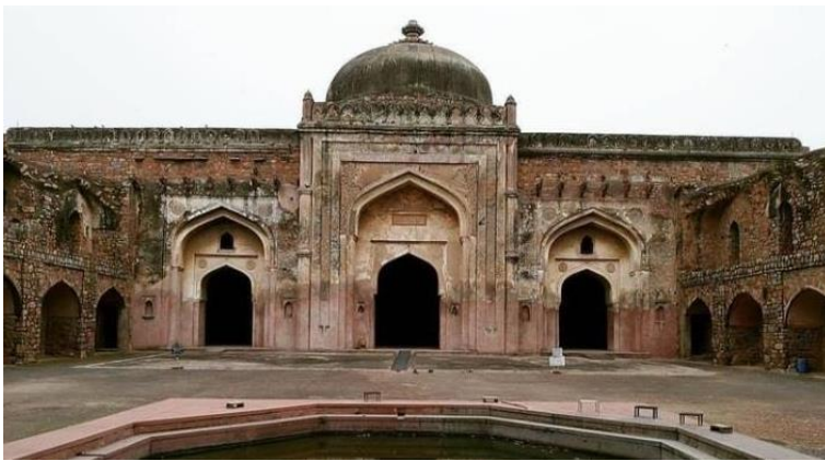
Fig. 7. Extensive algal growth is seen on the façade wall of the Masjid. Photo credit: Anas Khan - unzip_delhi
