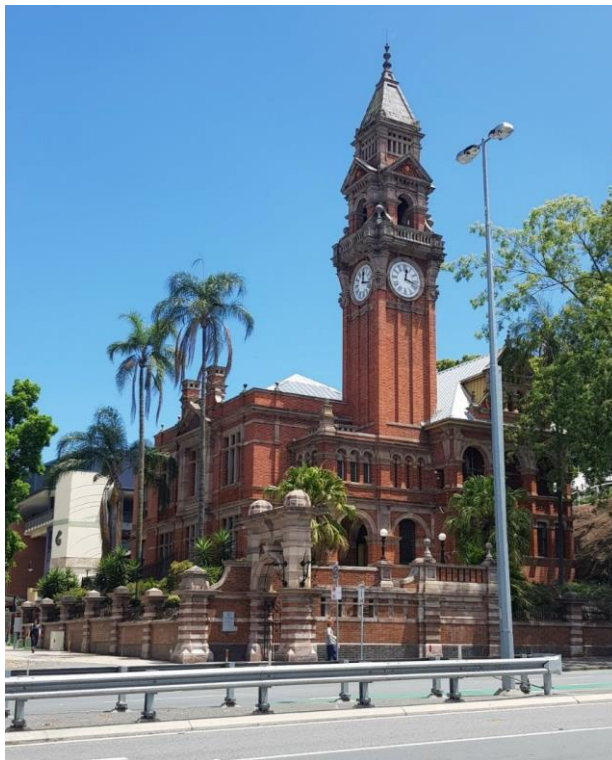
Fig. 4. South Brisbane Municipal Chambers
