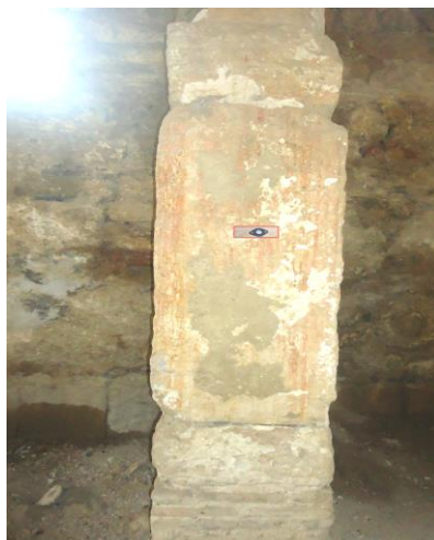
Fig. 7. The thermo-hygro-button location.
