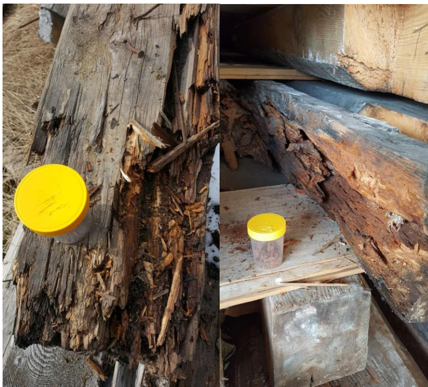
Fig. 3. Microbiological testing sample collection sites with visible alterations showing signs of biodeterioration.
