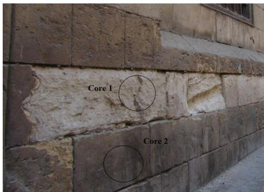
**Fig. 3.** Damage patterns (loss of surface and crumbling) which noticed in the north-west outdoor facade
