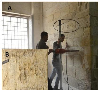
**Fig. 4. A** - general view of indoor facade with rising damp and **B** - close view of the marked area showing flaking of limestone surface
