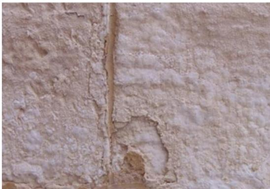
**Fig. 2.** The development of salt crystallization observed in the eastern outdoor facade with scaling of the outer surface
