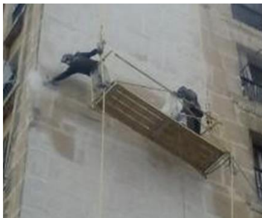
Fig. 7. Rehabilitation work on the Diar El Mahçoul tower in 2018
