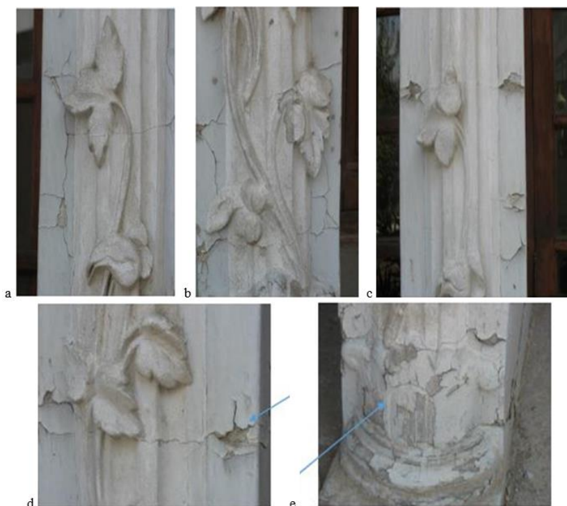
Fig. 1. Images of the stucco: a and b - cracks in the Abyaz House's column; c - erosion in the column; d and e - stucco falling and cracking at the base of a column.
