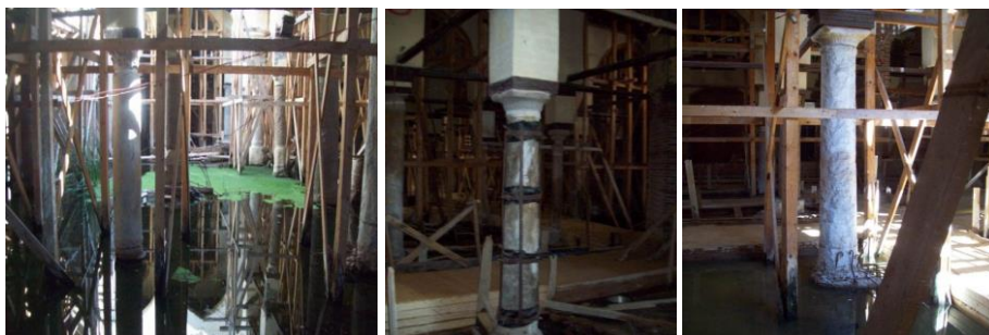
Fig. 2. Degradations and deteriorations of columns: left - ground water rising above the surface of the earth and the growth of algae within the mosque; center - staining and of soot layers cover some of the marble columns; right - intensive erosion of the surface layer
