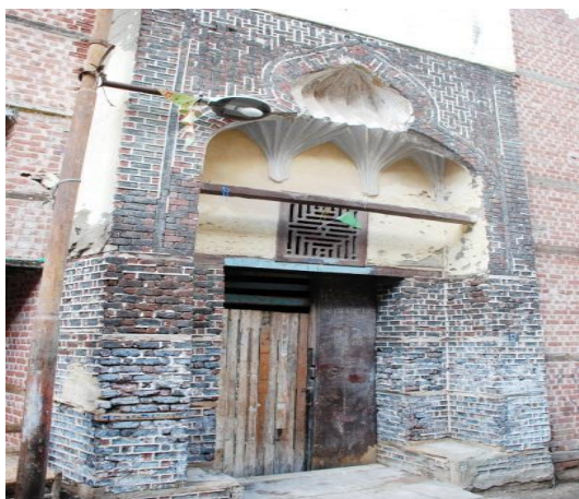
Fig. 1. The present state of preservation of the main entrances of Al Mahalli Mosque. rick disintegration due to the ground water rise and salt accumulation is obvious
