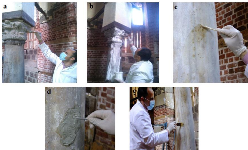
Fig. 16. Cleaning and consolidating process process of the marble columns: a - dry cleaning; b - salts removal process using poultices saturated with mild detergents with a low-pressure (900 psi) water rinse; c - final step, staining removing with detergents; d - repointing of the pits and gaps inside the marble columns; e – consolidating with Nano restore with 50% with acrylic materials with 50% concentration and dilute in water by 1:1 ratio agent time
