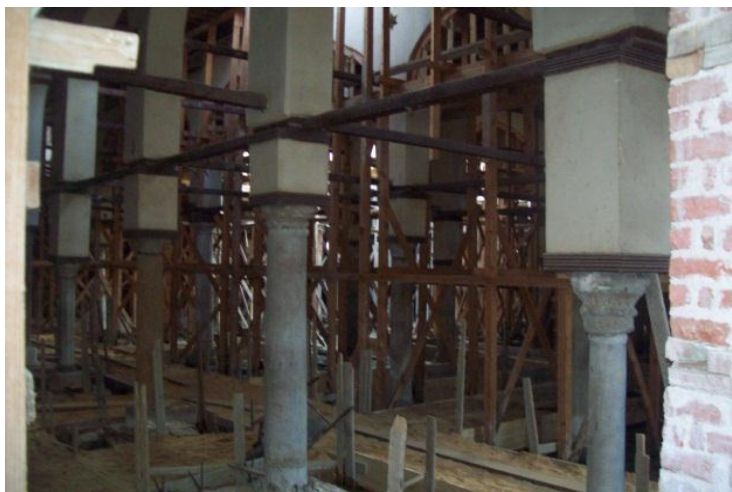
Fig 3. The pillars of the mosque and its abyss show signs of deterioration and imbalanced
