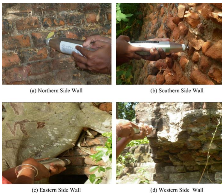
Fig. 1. Performing NDT using Rebound hammer at Karunguzhi Fort walls
