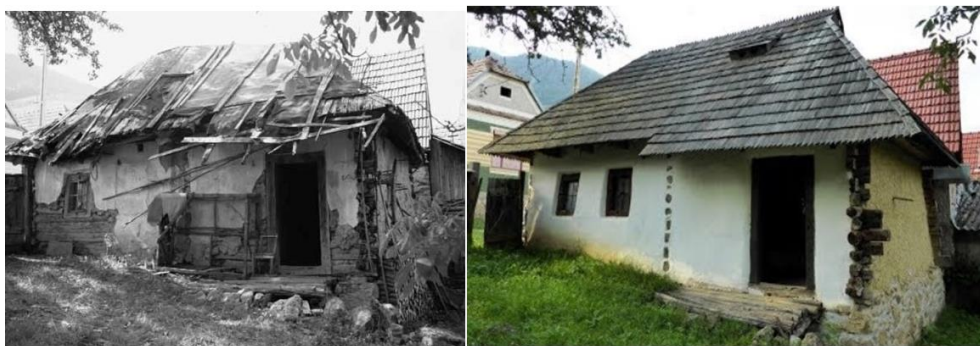
Fig. 3. The oldest dated rural house discovered so far in the Carpathian Basin, no. 260 from Rimetea (construction year 1668), photos taken by arh. Árpád Furu before and after the rehabilitation [1]
