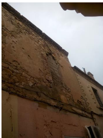
Fig. 12. The bad situation of the colonial constructions, suppression of a window
