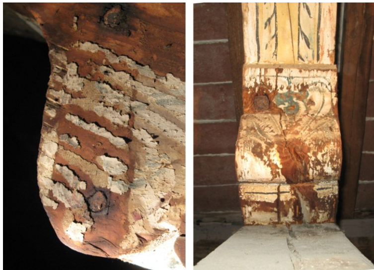
Fig. 2. Example of fabric on structural timber. Left: strip of fabric, residual on earlywood, to cover two nails. Right: end-grain of a cantilever with fabric (still present, with gaps) to upholstery nails and a shrinkage fissure
