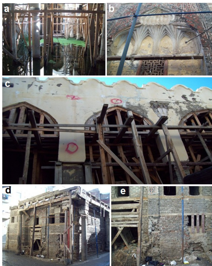
Fig. 3. Deterioration issues: a - Ground water rise inside Al Mahalli mosque; b - Deterioration due to rising humidity; c - Major arcades and the overhanging structure. cracks and fissures in the vertical walls; d - The main facade of El Manadily house, dangers cracks appeared in some pillars and separation between the façade and the radial walls; e - El Manadily house, deformation of the brick in the zone of the borders and main wall of the facade
