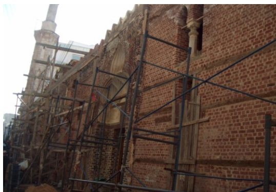
Fig. 2. The main and east facade of Al Mahalli mosque, under restoration and intervention processes.
