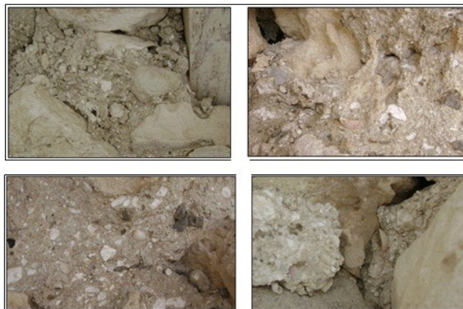
Fig. 9. Show decay of the mortar used
