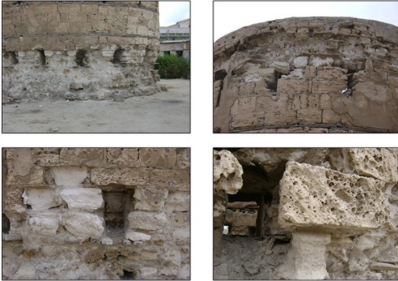
Fig. 2. Examples of deterioration phenomena in the military tower
