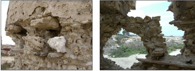
Fig. 8. Rapid decay to limestone blocks and collapse of whole sections of the wall
