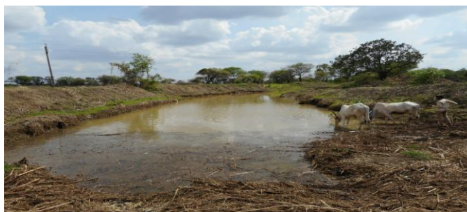
Fig. 8. Widened Nala (Drainage) in Awargaon village of Dharur sub-district in Bid district. Source: Picture taken during field visit
