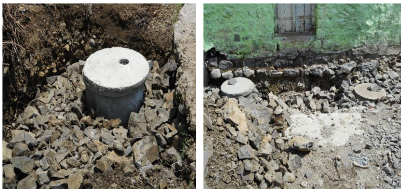
Fig. 6. Construction of Sosh Khaddas (Soak Pits) going on in Awargaon village of Dharur sub-district in Bid district. Source: Pictures taken during field visit
