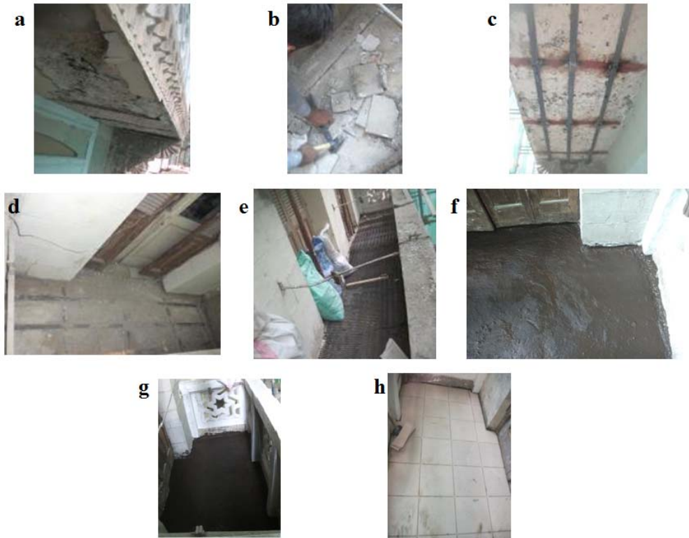
Fig. 15. Main steps in the intervention in the balcony floor: a. dismantling of the decorative units; b. Removing the old tiles; c. Strengthening of the steel beams using longitudinal and transversal steel plates from bottom; d. Strengthening of the steel beams using longitudinal and transversal steel plates from top; e. Adding steel mesh from top; f. Pouring cement mortar above the steel mesh; g. Adding water insulation above the cement mortar; h. Adding the sand, cement mortar and the ceramic tiles
