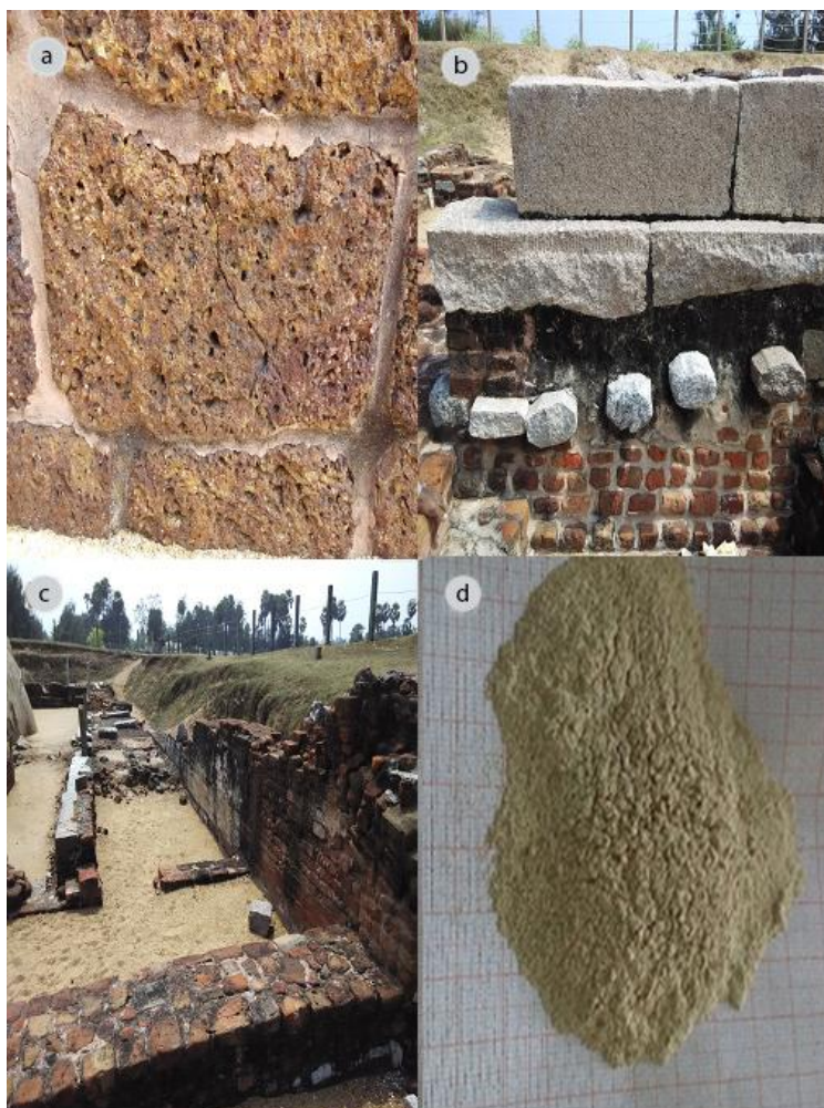
Fig. 2. Images of the Salvankauppam Temple and sampling areas: a. Laterite block with bedding lime mortar; b. rebuilt portions with granite stones; c. another view of remains of Temple; d. lime mortar sample
