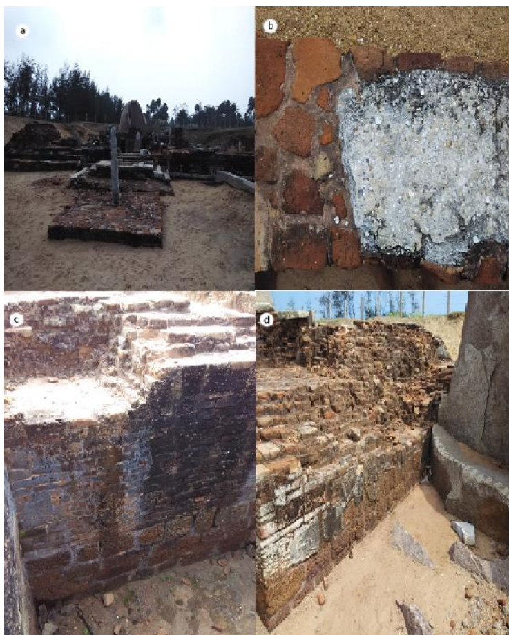
Fig. 1. Images of the Salvankauppam Temple and sampling areas: a. rediscovered; b. sea shells as aggregate in mortar; c. Laterite wall at bottom; d. brick work at top
