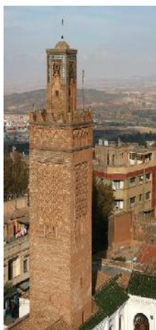
Fig. 1. Minaret of the Great Mosque before the restoration
