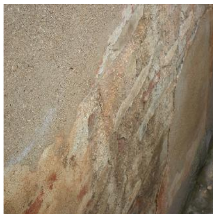
Fig. 8. Detachment of cement coating
