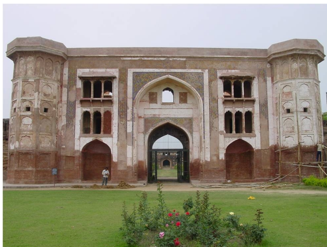
Fig. 1. General View of Dakhni Sarai, Jalandar, Punjab, India
