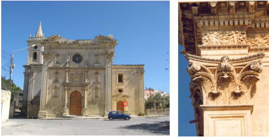
Fig. 1. The Church of Santa Maria; the location of the spring which is covered by this study is indicated in red (left) and a well weathered acanthus capital (right)
