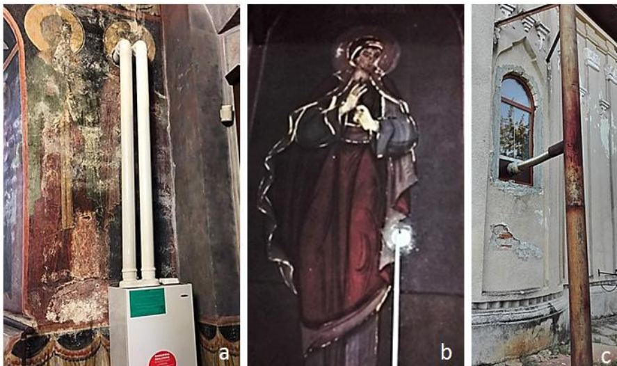
Fig. 6. Inadequate installation of heat and power systems inside of the historical monuments:
