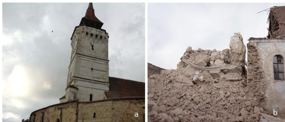
Fig. 8. The Tower of the Evangelical Fortified Church, Rotbav , Brasov: a. The church tower before collapse; b. The church tower after collapse [Photo source: a. Țetcu Mircea Rareș , 2013; b. http://tinyurl.com/j5tre9g ]
