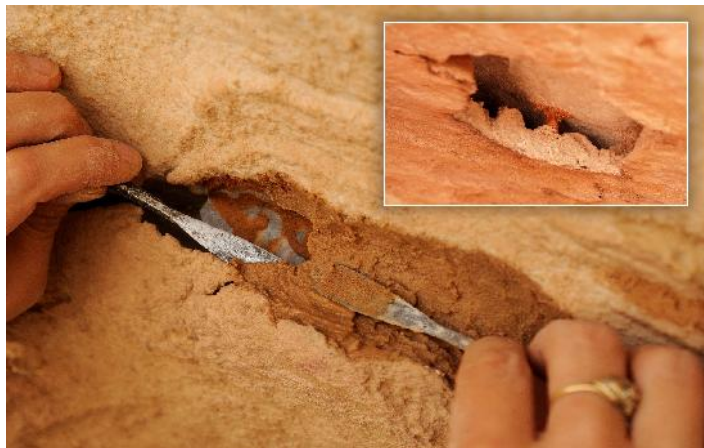
Fig. 13. Cave of Swimmers. Sealing of openings and cracks
