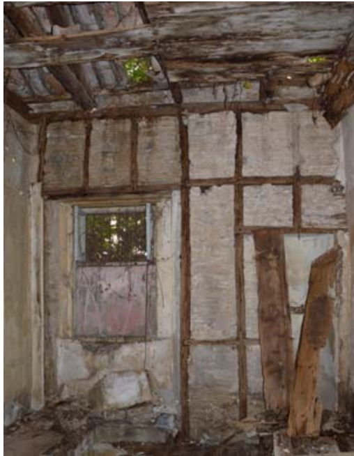
Fig. 2. An example of Borbone constructive system, masonry reinforced with an inner timber framing.
