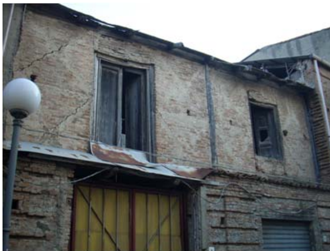
Fig. 4. Seminara (Rc). The consistency loose of the inner wooden member has generated on the brickwork 45° degree cracks tracing precisely the saint Andrew crosses.
