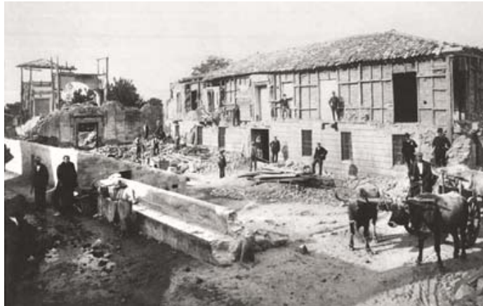
Fig. 6. Messina. A baraccato building characterized by the overturning of the external masonry leaf after the 1908 earthquake.
