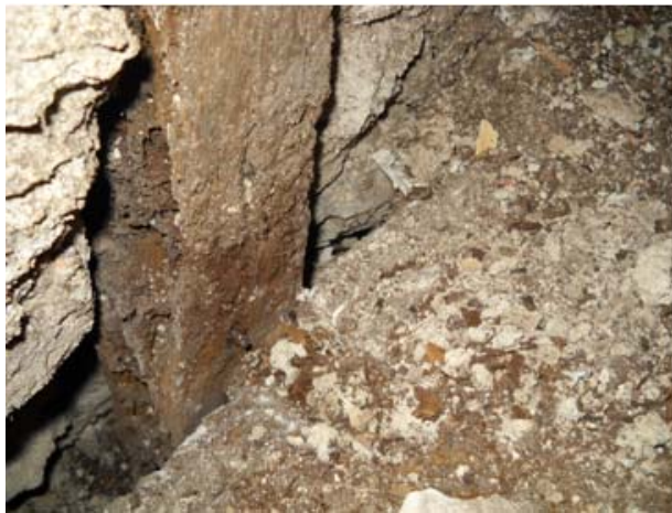
Fig. 3. A decayed wooden post of a frame in which the damaged timber is reduced in powder.
