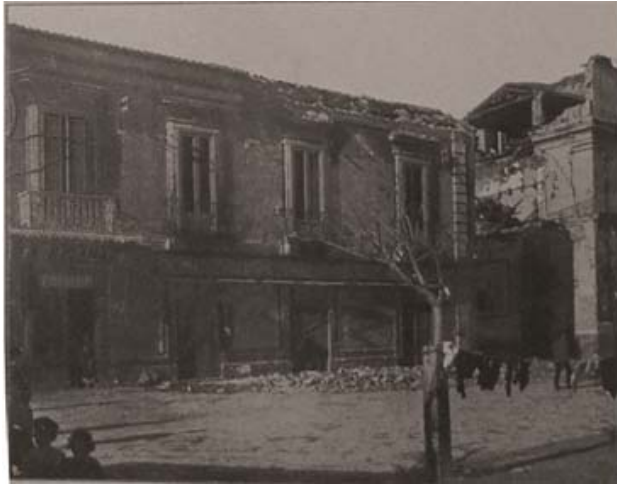
Fig. 5. Reggio Calabria. A baraccata building damaged by the 1908 earthquake.
