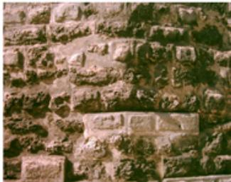
New additions used for restoration of the Nymphaeum with different materials like limestone blocks and cement mortar
