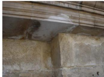
Efflorescences formed on the surface of the new stone added to Nymphaeum.
