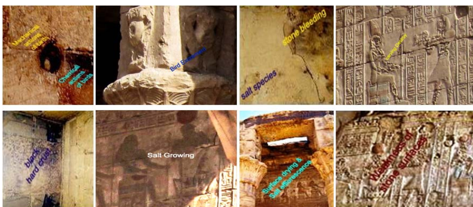
Fig. 2. Showing some deterioration patterns affected sandstone of Edfu Mammisi
